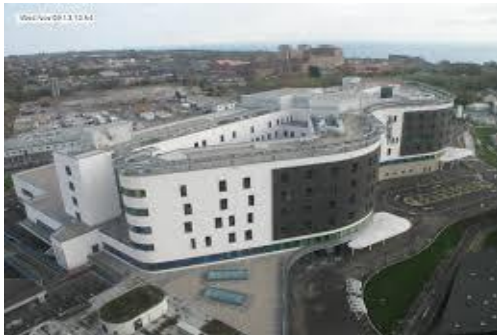
Royal Victoria Hospital, Kirkcaldy, VK Trend BMS, Gent Fire Alarm
